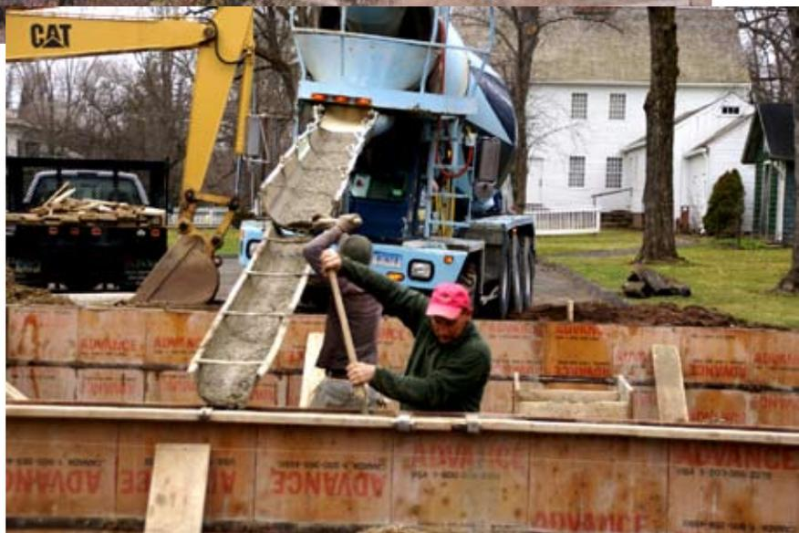
*Top: The Society's "new" old barn, shown here before it was fully disassembled in Canada, is being erected at the King House Museum. Lower: As concrete is poured for the new barn foundation, Doug Colson spreads the mix along the form as Brandon Stafford encourages the flow from the trough.*
