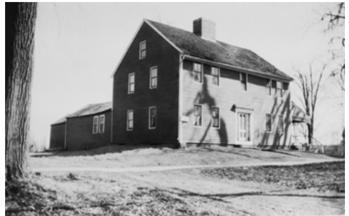
The Alexander King House before renovation by Samuel and Helena Bailey Spencer, 1926
